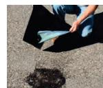
4. Cut patch to extend beyond repair area by 4" on all sides. If 2 or more pieces are required to cover the area, a min. of 3" overlap is required.
