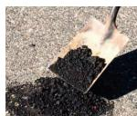
1. Remove loose material from repair site. Fill and seal intersection cracks around repair. Fill area with hot or cold asphalt fill mix.
