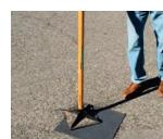
5. Peel the release film - apply to prepared area. Tamp or roll to bond patch to clean, dry pavement. Patch should be exposed to traffic immediately.
