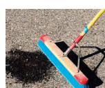
3. Clean area of dust, debris, salts or oils. Dry completely. If ambient temp is below 75°F, either apply propane torch to surface and heat or apply approved primer.
